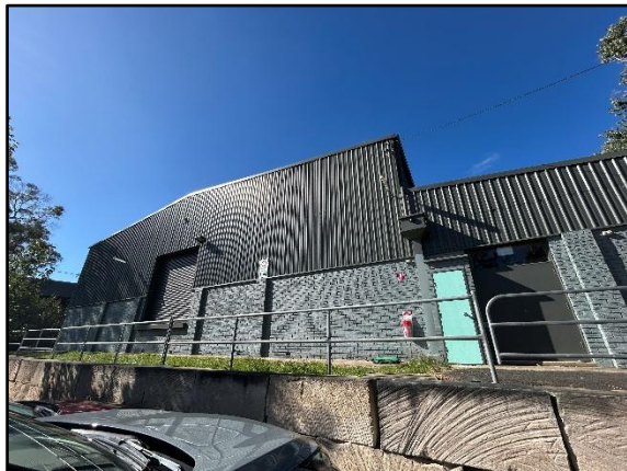
Figure 39. External view to the northern façade of McGrath Hall, facing south.
