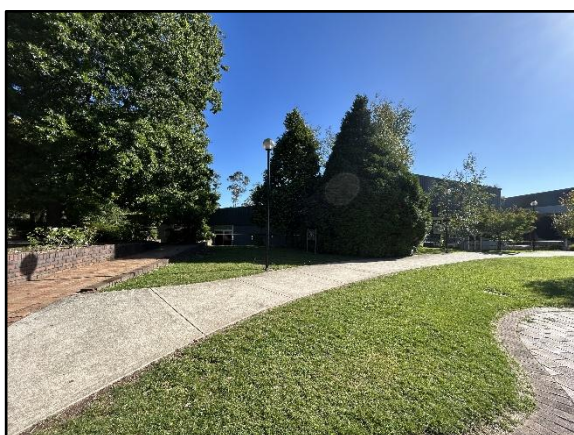
Figure 45. External view to the southern façade of McGrath Hall and planting along the southern elevation, facing north.
