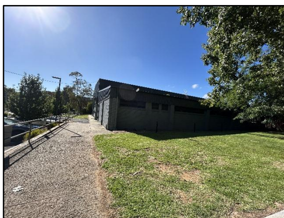
Figure 46. External view to the north-western corner of McGrath Hall, facing east.
