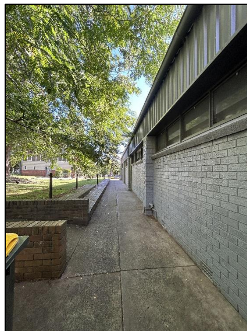
Figure 42. External view to the western façade of the building, concrete walkway and brick-masonry retaining walls, facing north.
