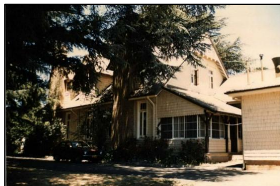
Figure 27. Western elevation of Riversdale House, 1991, showing new additions (Source: Wingecarribee Shire Council Heritage Study, 1991, Part A, Ref. No: W10189, p. 20).
