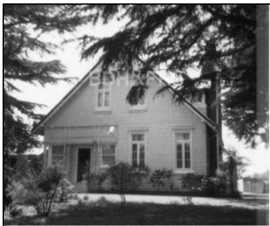
Figure 24. Front elevation of Riversdale House, indicating that the front veranda had been enclosed and the timber cladding painted, 1979 (Source: Berrima District Historical and Family Society, Image: 106962).
