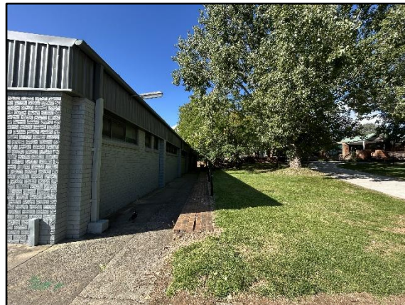
Figure 40. External view to the western façade of McGrath Hall, brick-masonry retaining walls and mature trees, facing south.
